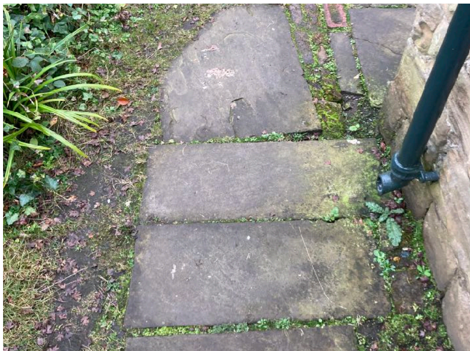
Figure 06: The existing down-pipe, discharging onto the footpath. The stone flags in this area often become slippery due to algae buildup on the wet flags.
